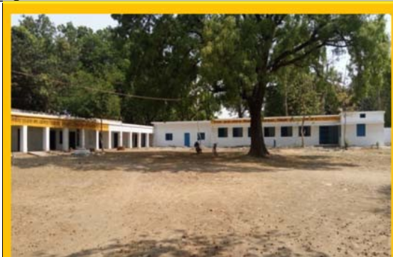
Renovation of Hr. Sec. School at Sijahata
